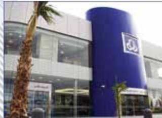
Al-Rajhi Bank (External)
