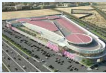
Khaleej mall (Under construction)
